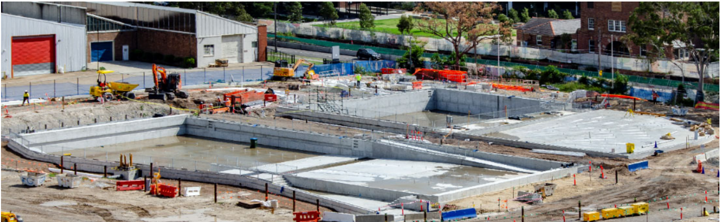
Gunyama Park Aquatic and Recreation Centre: Construction works
